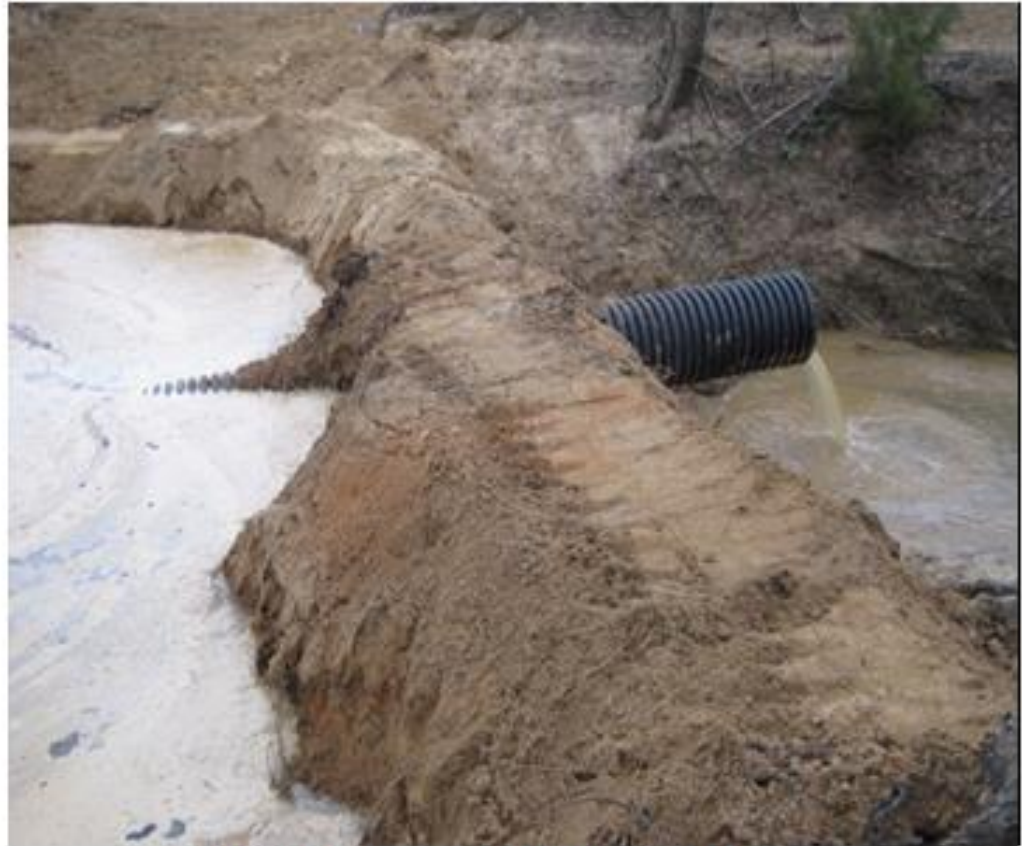
Finished emergency flume dam # 3.
